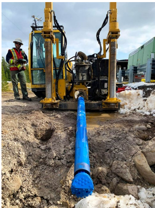
Figure 3.2: Horizontal Directional Drilling Midi Rig
